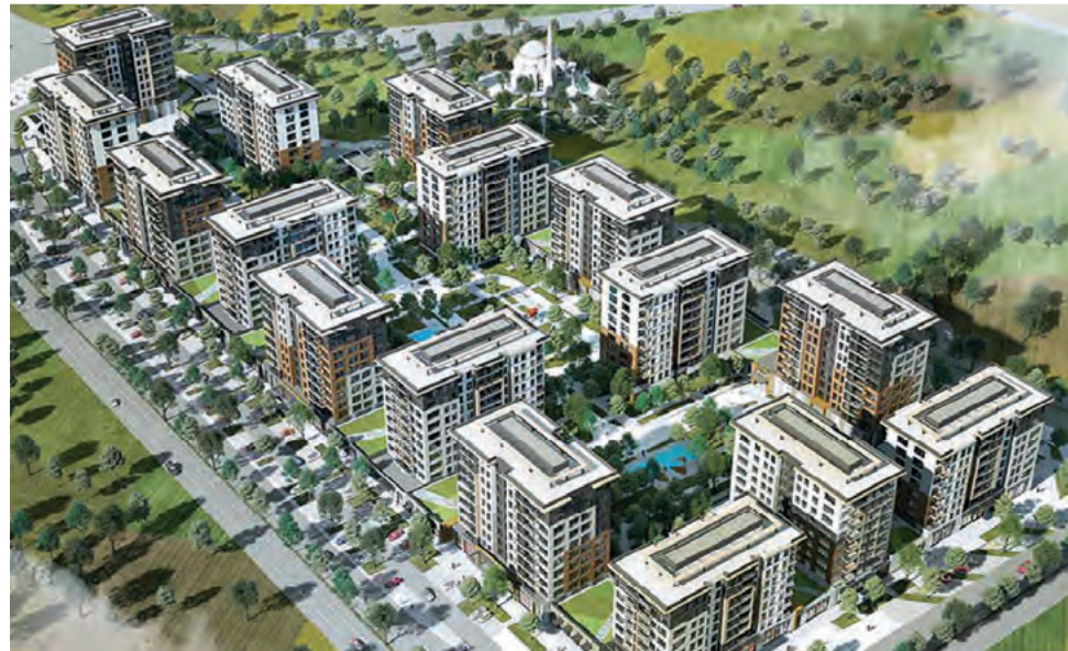
The residential real estate project Mavera Comfort in Başakşehir Istanbul was completed in 2023.
